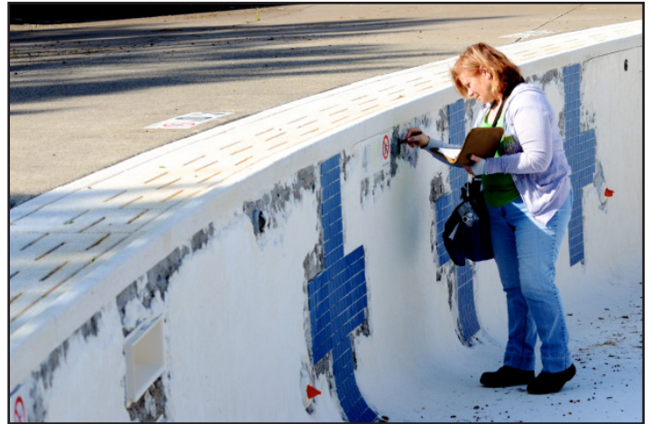
Verhoef inspects the Sellwood Pool in NE Portland.
